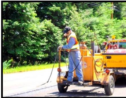
Cam Jones spraying tack oil for our grind and pave project that we did on Hwy 19A in Courtenay, with Oliver overseeing the activities. The
