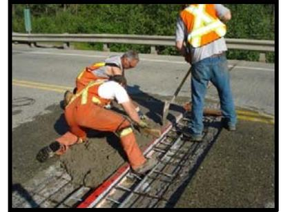
Below—One of the new sidewalks we fabricated has been installed on Simms Creek Bridge in Royston. This is the site of a new bike and walking path which will extend from north of Courtenay eventually to Buckley Bay Ferry.
